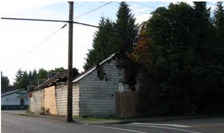
Figure 2. Former Warehouse on property.
