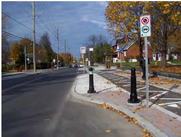
Figure 7: Pavement markings at bus stops with wide landing area
