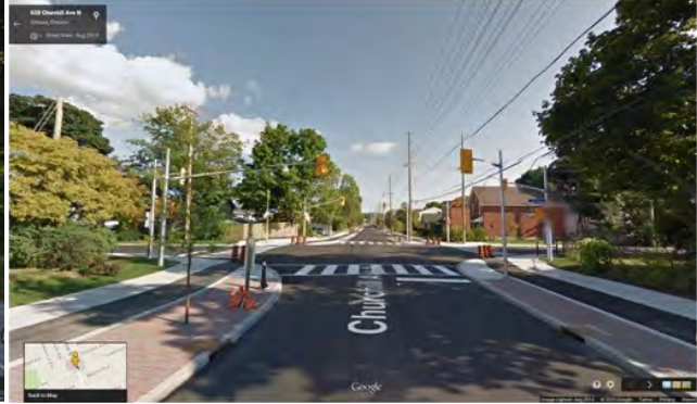
Figure 4: After – clear delineation of the cycling and pedestrian facility Source: Google image
