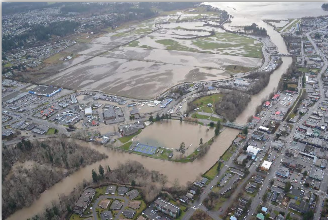
Photo 1: City of Courtenay Flooding December 2014
