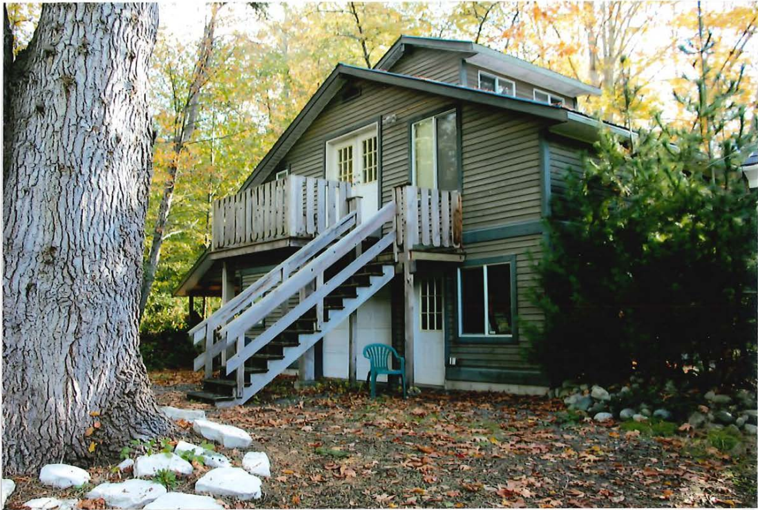
View of Shop/Suite showing south side of building
