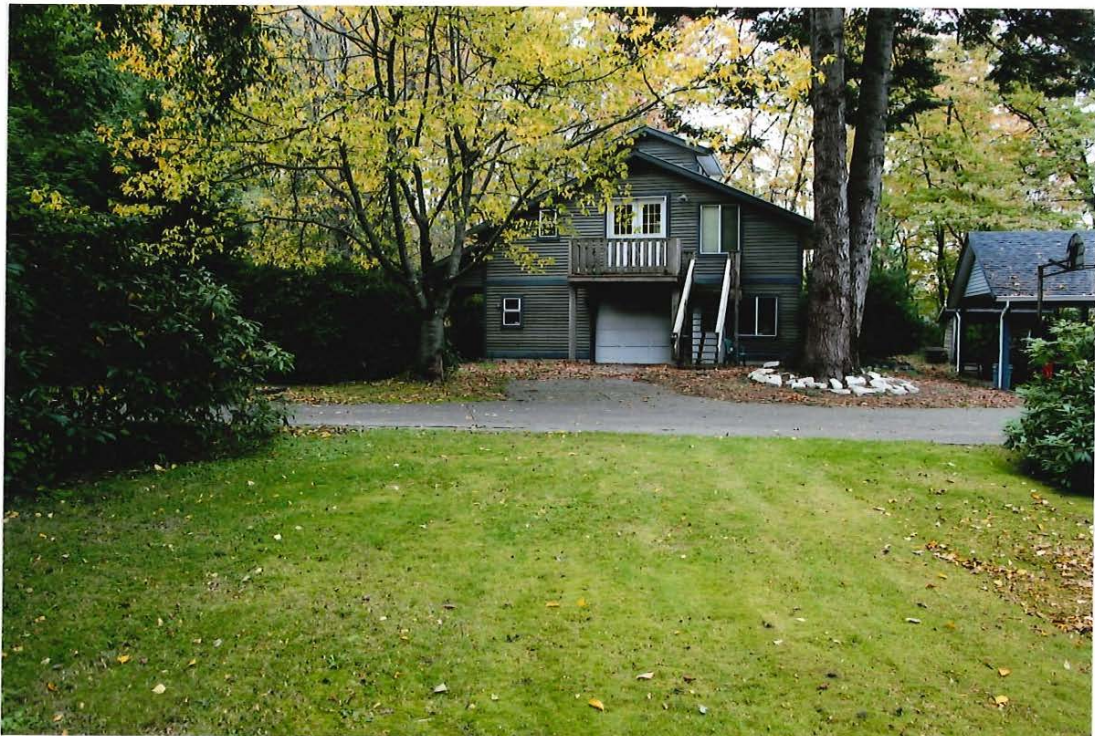
Front view of Shop/Suite showing proximity to yard and Main Home
