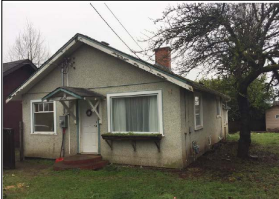
Figure 4. View of existing building front yard façade.
