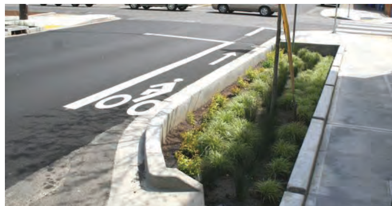
A bioretention planter captures runoff from a sidewalk or street and allows it to feed vegetation and infiltrate into the soils below.
