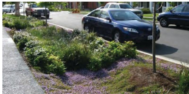
A vegetated swale conveys, treats and infiltrates runoff from adjacent sidewalks and road surfaces.
