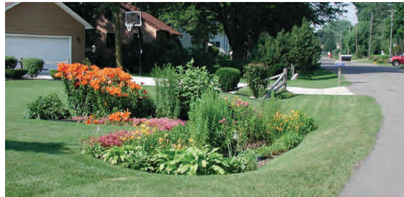
Rain gardens use plants and permeable soils to store, filter, infiltrate and evapotranspire stormwater runoff.
