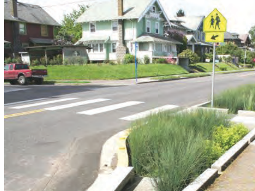
Curb extensions and planted swale provide safe pedestrian crossing.
