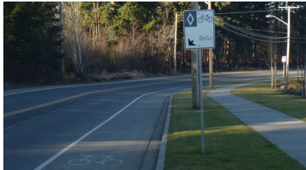
A collector road with a dedicated cycle lane and sidewalk provides access to nearby amenities.
