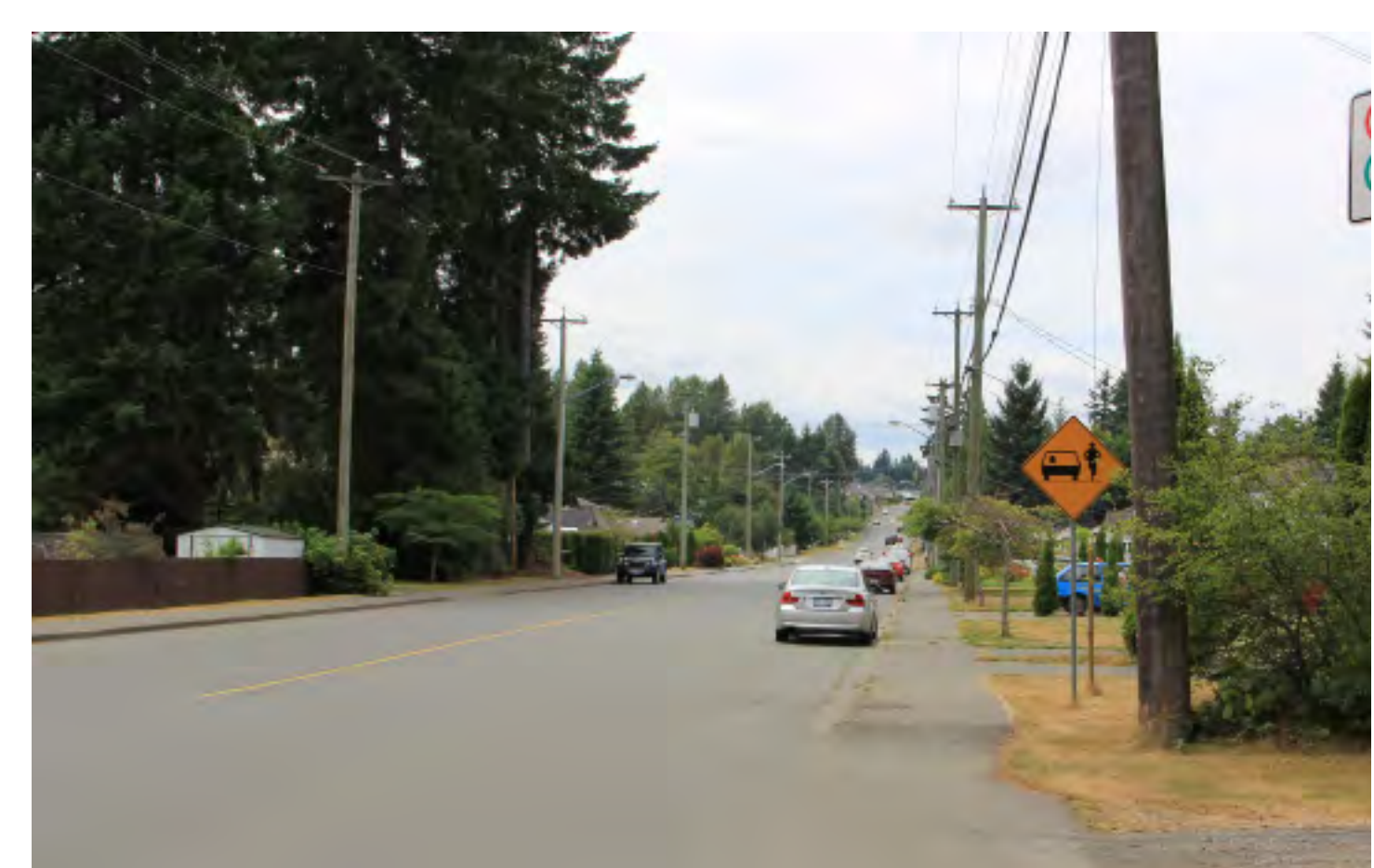
1st Street Shared On-Road Cycle Lane
