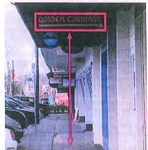
The distance between the bottom of the sign and the sidewalk below is referred to as clearance
