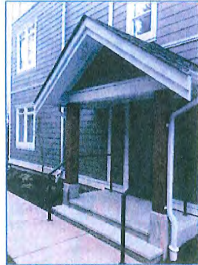
Figure 4 - Secondary entrance detailing
