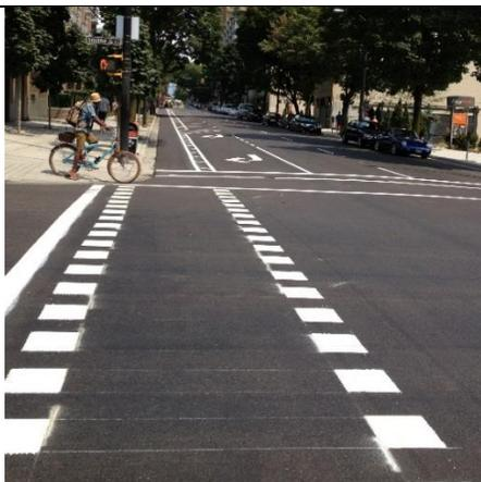
**Crossbikes and elephant's feet** are pavement markings that indicate a crossing zone in which a cyclist does not need to dismount. They may be combined with a pedestrian crosswalk or may be used to indicate a separate bicycle crossing.
