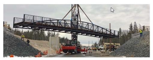
Figure 6: Installation of a Bowstring Truss Bridge
