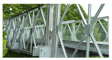
Figure 19: Modular Bridge Protective Screen System
