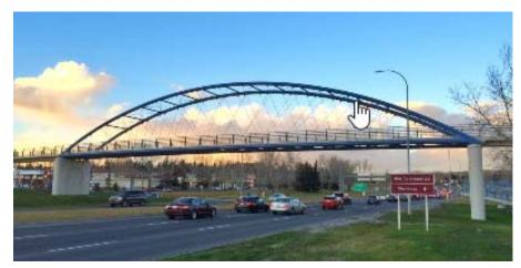
Figure 10: Network Arch Pedestrian Bridge Example
