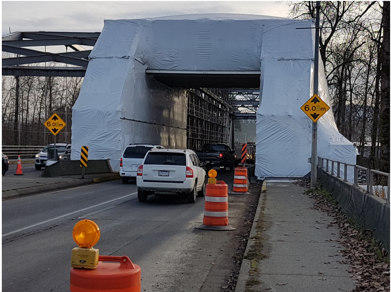
Figure 1: Fully Wrapped Bridge Accommodating Traffic
