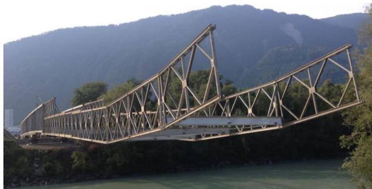
Figure 36: Truss being push-launched with launching nose attached
