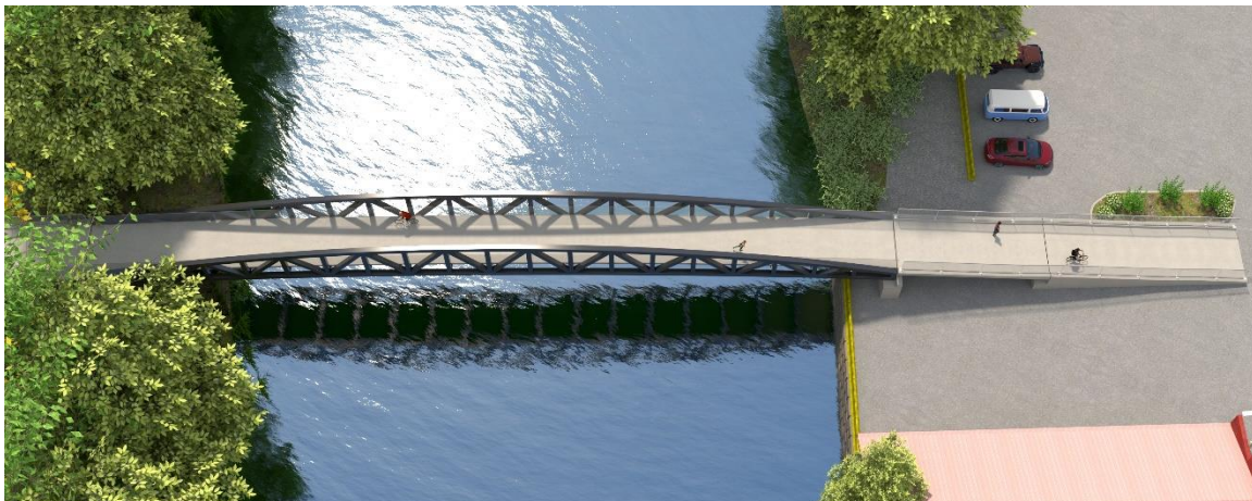
Figure 30: Bird's eye view of pre-engineered bowstring truss option at proposed project location
