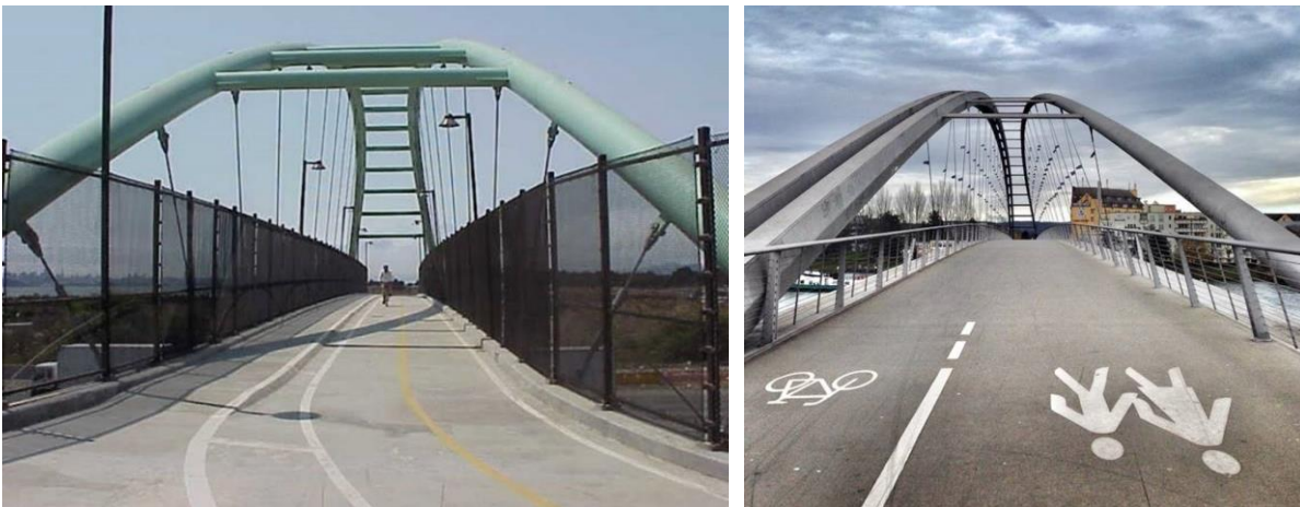
Figure 52: painted delineation examples on 5.4m wide deck over I-80 (left) and 5.5m deck over the Rhine River (right)
