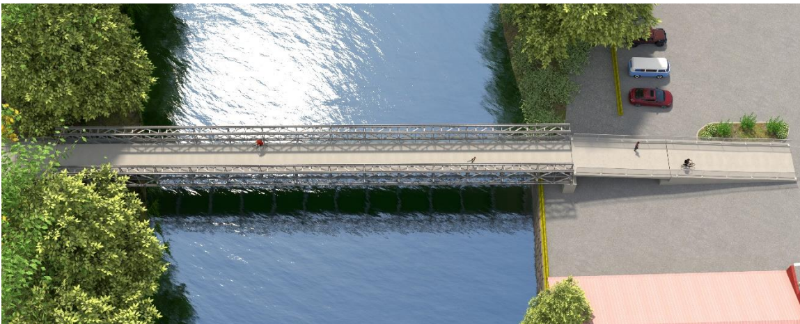
Figure 37: Bird's eye view of modular panel (Bailey) bridge option at proposed project location
