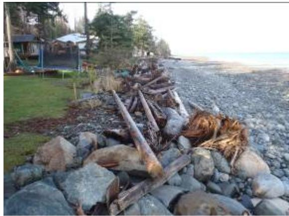
Shoreline armoring using conventional rip rap showing effects to neighboring property (top left) and restoration after using rooted tree revetment (top right). During Nov 24, 2011 storm (bottom left) and day after (bottom right).
