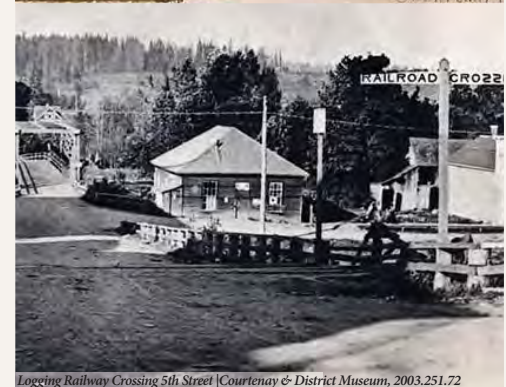
Logging Railway Crossing 5th Street | Courtenay & District Museum, 2003.251.72
