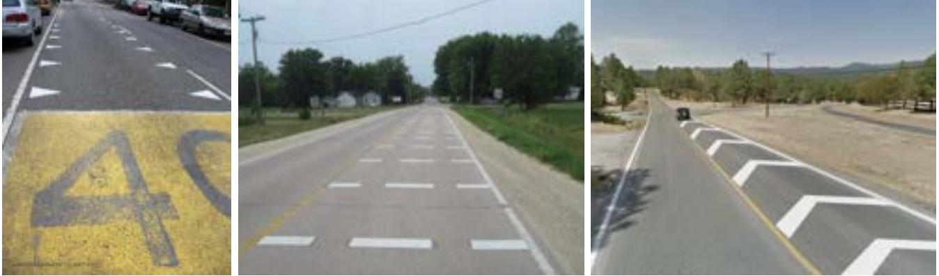
Figure 23. Sample Application of Transverse Lane Markings (Dragon Teeth – Left 36 , Transverse Bars 37 – Middle, Converging Chevrons 38 – Right)
