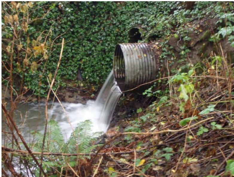
Photo 1. Example of a perched culvert installation (Glen Urquhart Creek at 10 th St. E.) acting as a barrier to fish migration and contributing to limited fish productivity in urban stream channels.
