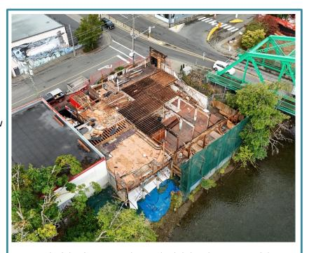
Removal of the former Bridge Nightclub has been a careful process to ensure protection of the river. Green netting prevents debris from falling into the water below.
