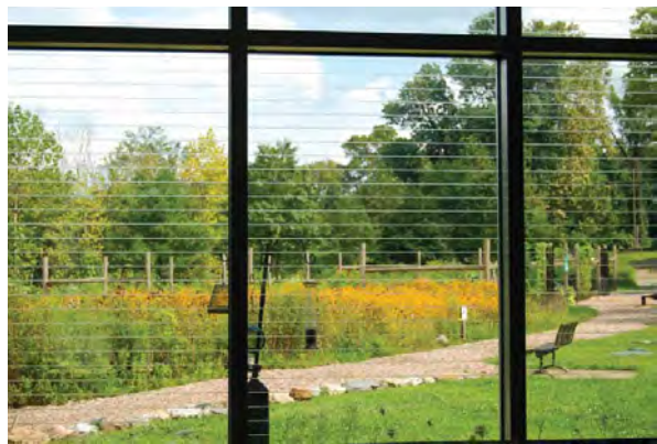
Example of bird-friendly glazing (guideline 28). The pattern shown is etched directly on lower-floor windows to reduce the frequency of bird collisions.
