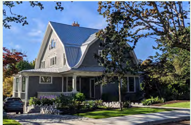
Example of a number of design elements such as gables, verandas, and decorative shingles incorporated into a single-residential home to create architectural interest (Additional Guidelines for the Old Orchard and Terminal Addition Neighbourhoods 5).
