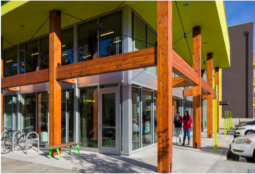
Example of using exposed mass timber structural elements as part of an emerging west coast character (guideline 23). Also includes pedestrian and cycling supportive features such as private sidewalks along the length of the building entry (guideline 57); weather protection (guideline 59); and seating and bike parking (guideline 31).
