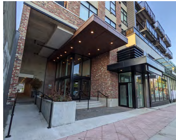
Example of a diversity of pedestrian-scaled visual elements being incorporated into the street-facing building façade (guideline 16). In this case a number of distinct building entries are incorporated.
