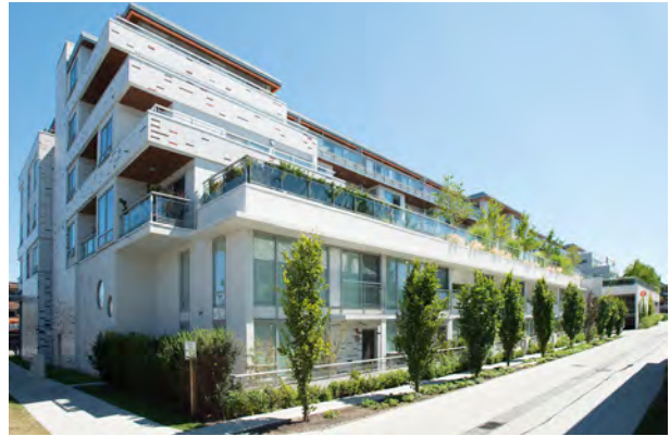
Example of stepped building massing and articulated walls to develop building form and character (guideline 12).
