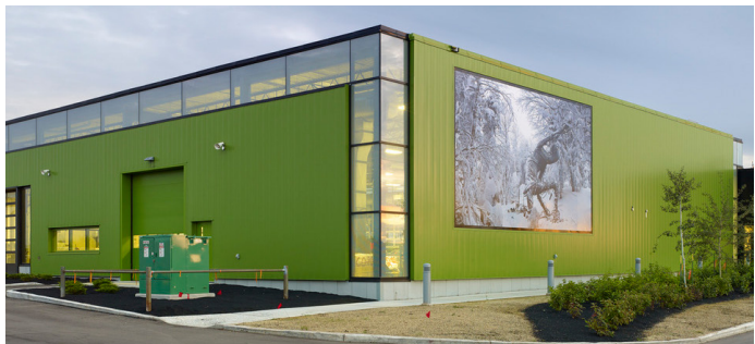
Examples of different forms of artistic treatments and landscaping to create visual interest along large expanses of unavoidable blank walls (guideline 26).
