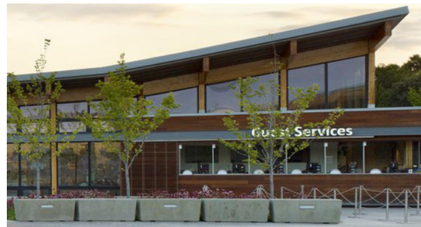
Example of stepped and varied rooflines to develop building form and character (guideline 12).
