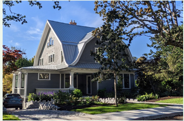
Example of a number of design elements such as gables, verandas, and decorative shingles incorporated into a single-residential home to create architectural interest (Additional Guidelines for the Old Orchard and Terminal Addition Neighbourhoods 5).
