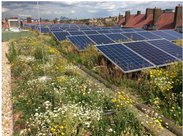
Example of solar photovoltaic panels being incorporated with greenroof elements (guideline 94 and 95).
