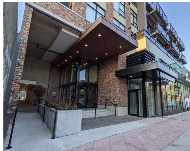
Example of a diversity of pedestrian-scaled visual elements being incorporated into the street-facing building façade (guideline 16). In this case a number of distinct building entries are incorporated.
