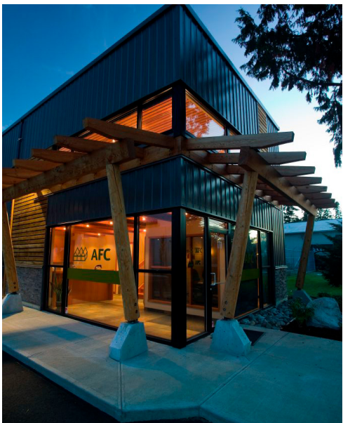
Example of an industrial building incorporating changes in exterior colours and textures (guideline 21); and wood with varied details and columns (guideline 22).
