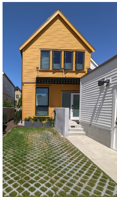
Example of a pervious driveway treatment to allow for rainwater infiltration (Landscaping 11).
